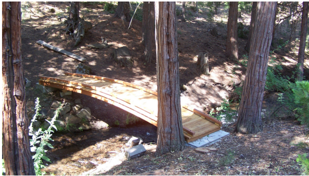
New Foot Bridge
